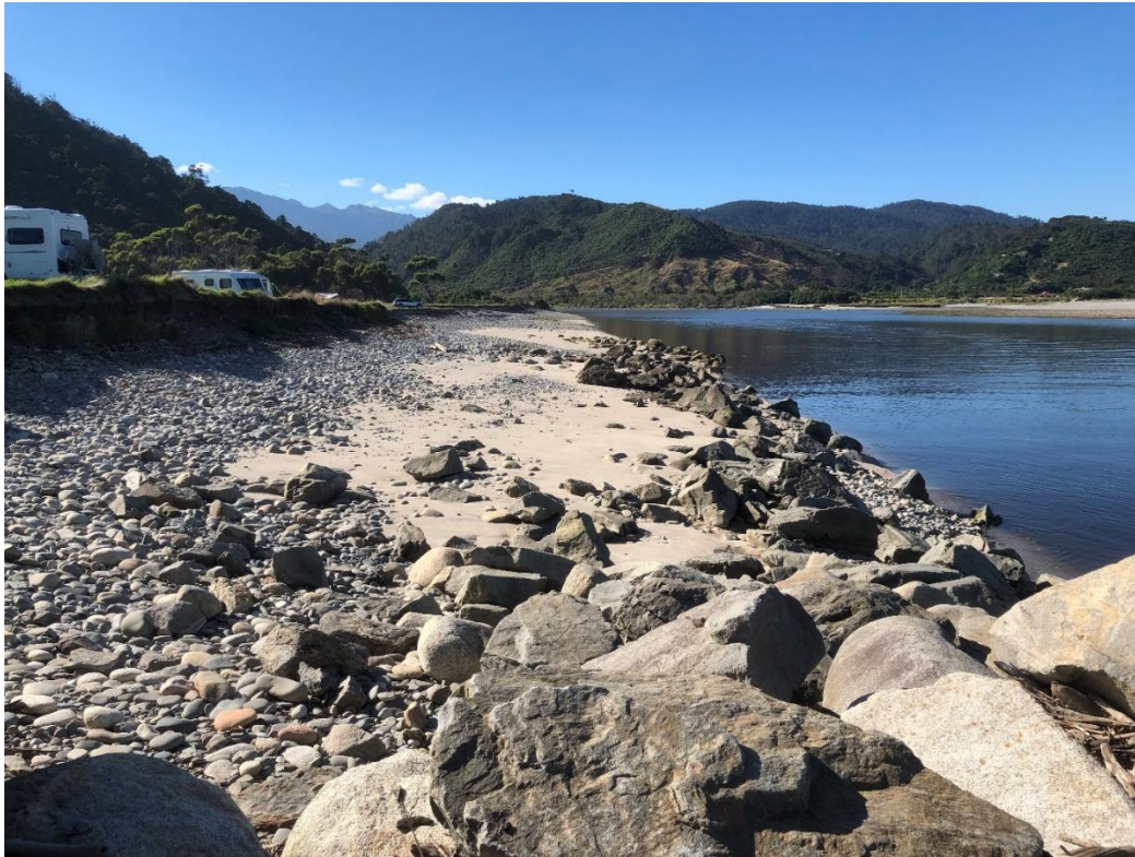
Figure 3-2: View upstream on north bank along remnants of training wall.
