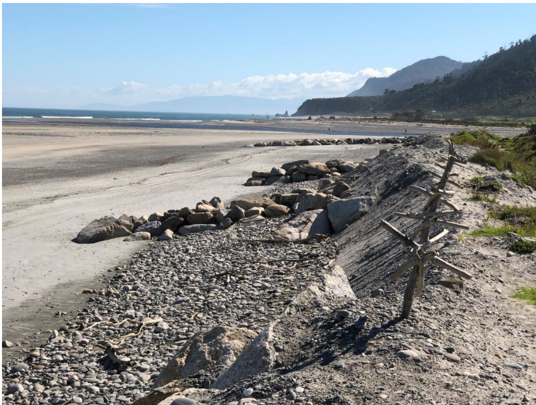
Figure 3-7: The 3 rd and 4 th stub groynes and the spit-tip groyne in the background. Note northward thickening of cobble ramp towards the nearest (3 rd ) groyne.
