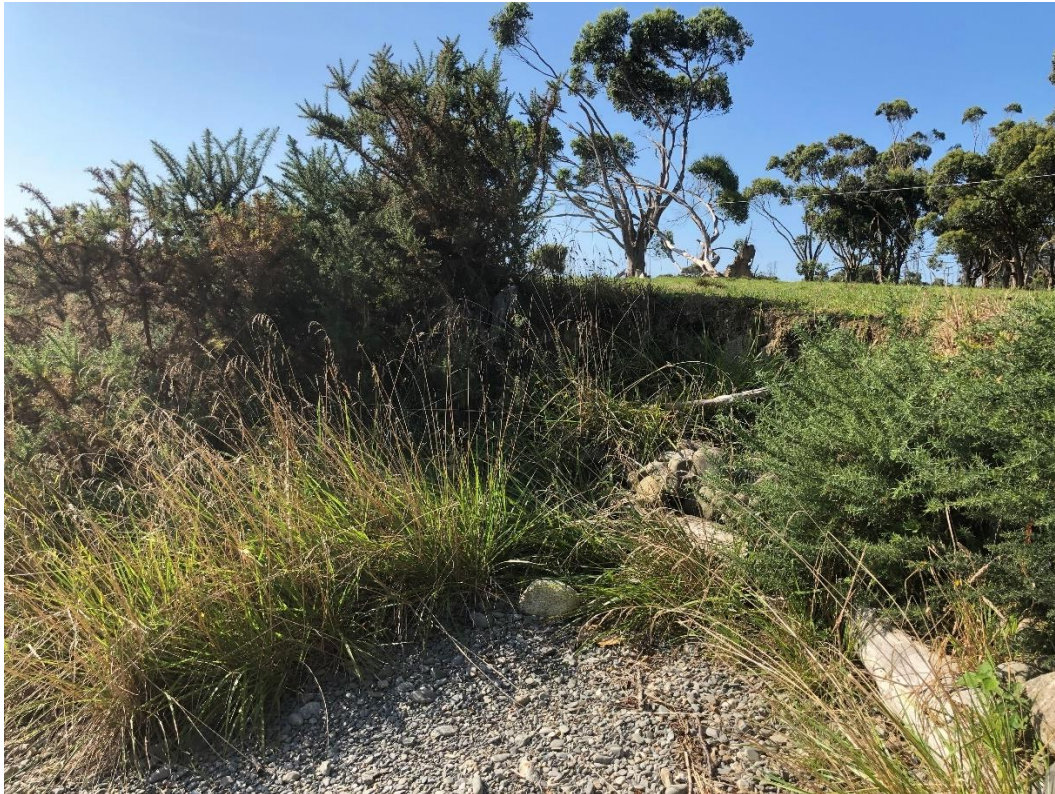
Figure 3-4: Close-up of vegetated-over erosion scarp between north bank stub groynes.
