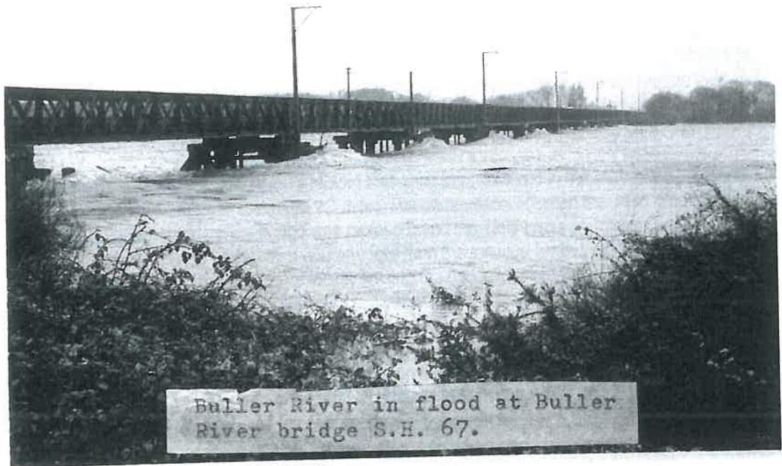
Photograph 2 - The 1970 Flood at the old Buller Bridge (taken from the left bank facing slightly downstream)
