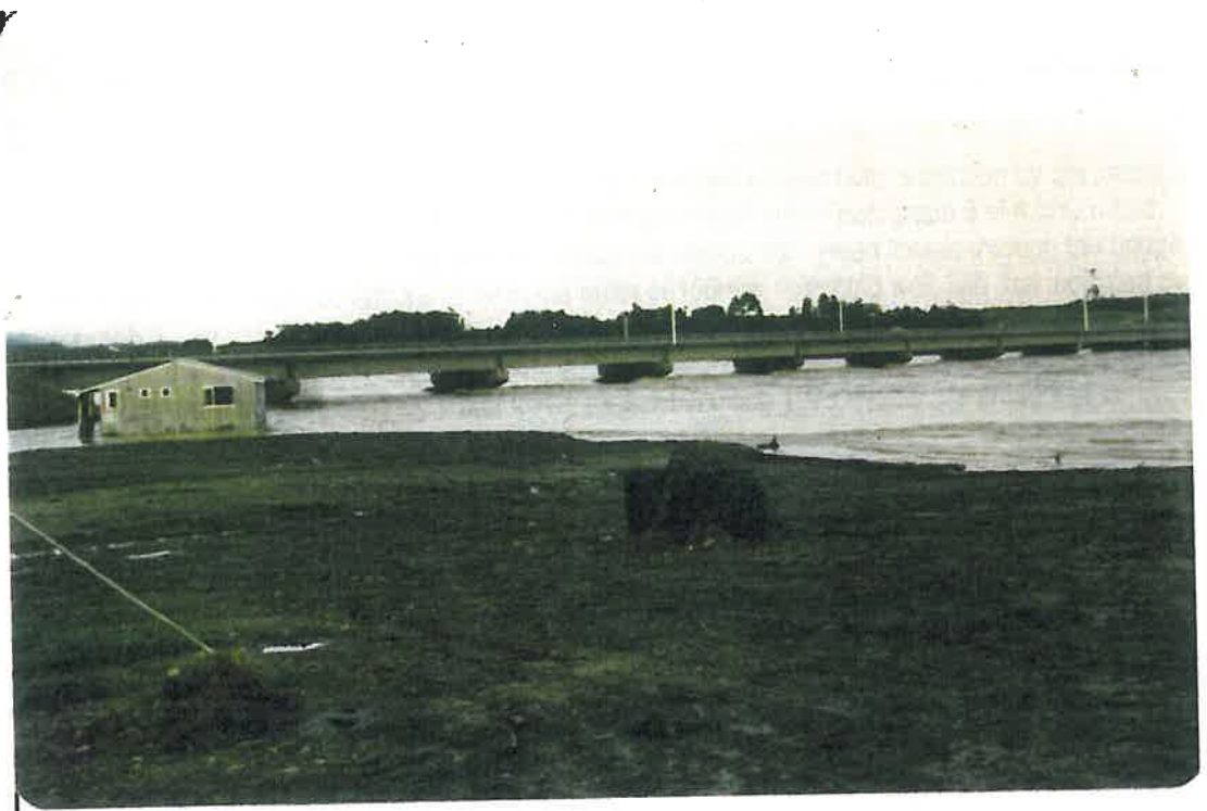
Photograph 3 - The 1979 Flood at the new Buller Bridge (taken from the right bank facing upstream)
