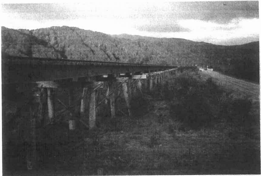
Photograph 1 - Railway Trestle Bridges Spanning the Orowaiti Overflow
