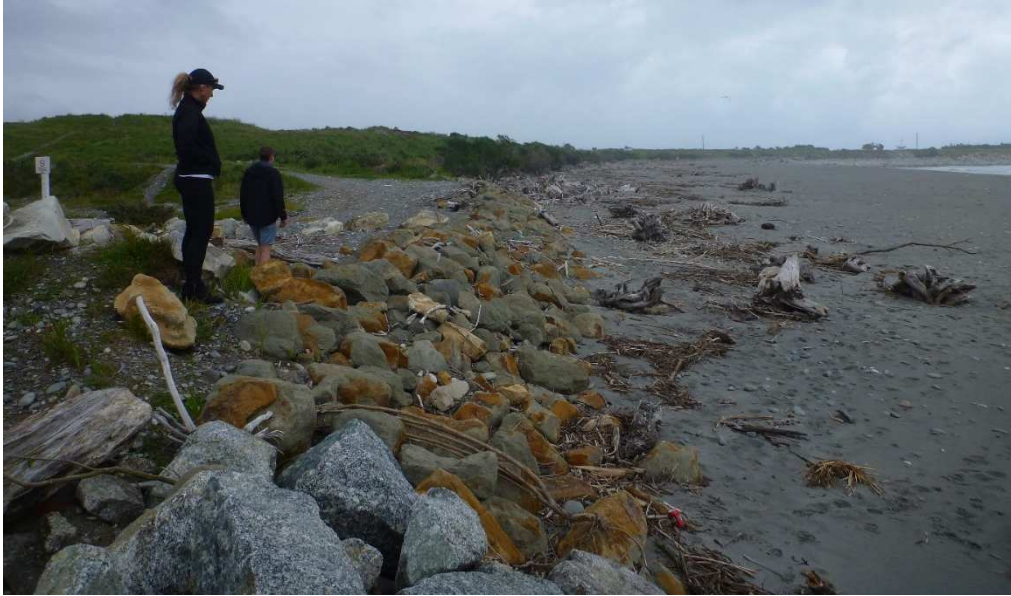
Figure 3-2: Rock extension south of the carpark to protect the Lagoon Cut entrance. [Credit: M. Hicks, 21/11/2017].
