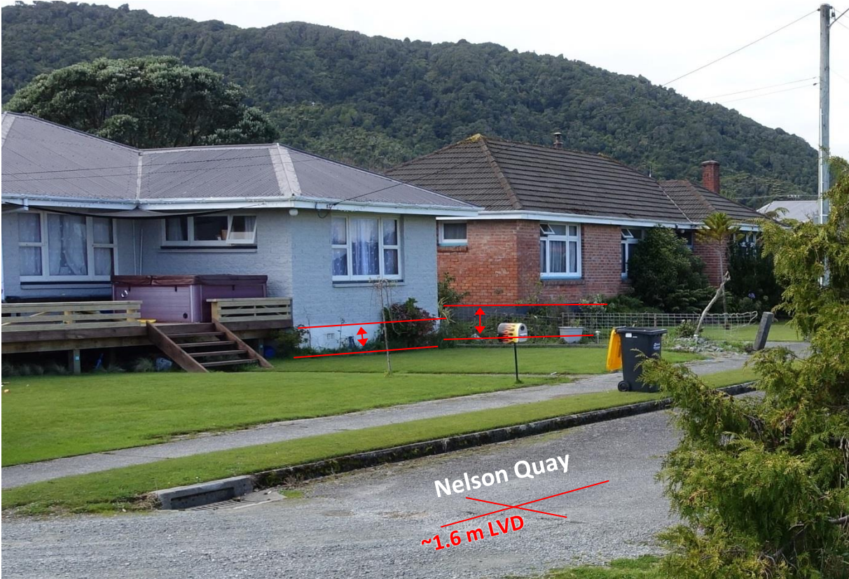
Figure 2-4: View eastwards from the north-western end of Nelson Quay. Raised floor levels and low level of road marked (from LiDAR) in red..
