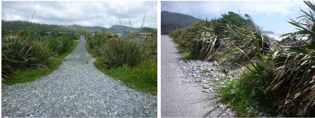
Figure 3-2: Continued overwash deposits onto Morpeth St (left) and Beach Rd near Statham St (right). [Credit: M. Hicks].
