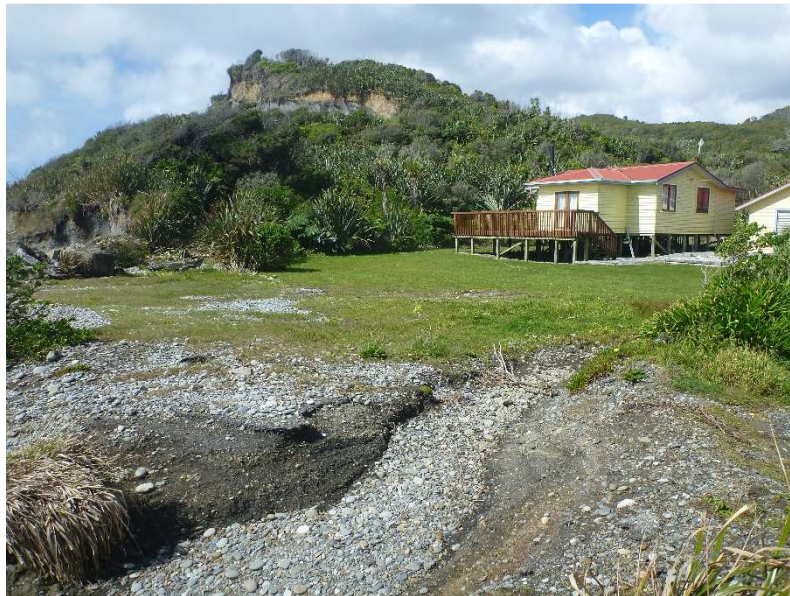
Figure 3-6: Relocated Forbes house, Holland St. Former foundations and driveway are just visible 20-25 m seaward (left) from house [Credit: M. Hicks].
