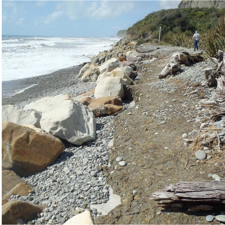
Figure 3-5: Current condition (21 November 2016) of the northern end of the rock revetment. [Credit: M. M. Allis].
