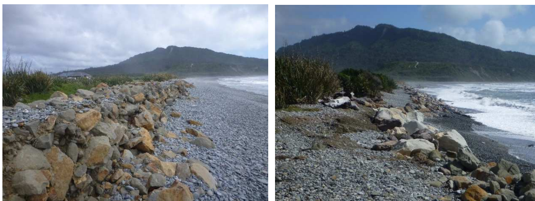
Figure 3-4: Continued beach retreat against rock berm (left) and along the entire foreshore (right). [Credit: M. Hicks].
