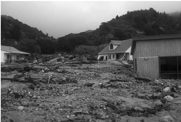
Figure 2 – Awatariki stream debris-flow fan, Matata, Bay of Plenty, New Zealand, May 2005; here a new subdivision was in the process of development to its full potential (McSaveney et al. , 2005).
