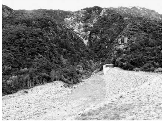
Figure 11 – Debris-flow deflector wall (right) at Glencoe Stream, Aoraki/Mt Cook. Note debris-flow terrace (from 1957 event) on far side of stream. A larger, older terrace is hidden in the trees behind it.
