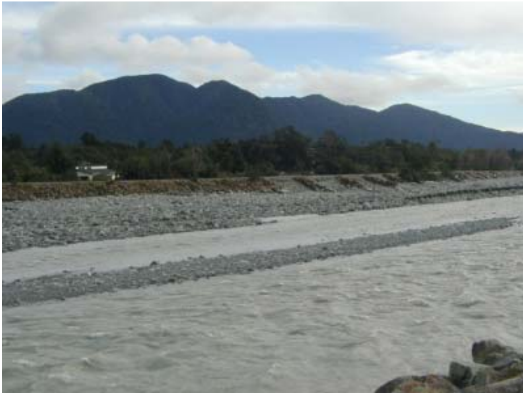
Figure 5.2: Holiday Park stopbank. The top floor of a building at the Glacier Gateway Motel is visible above the stopbank at the left (white), and the roofs of several of the motel units at the Black Sheep Lodge are visible near the middle of the picture.
