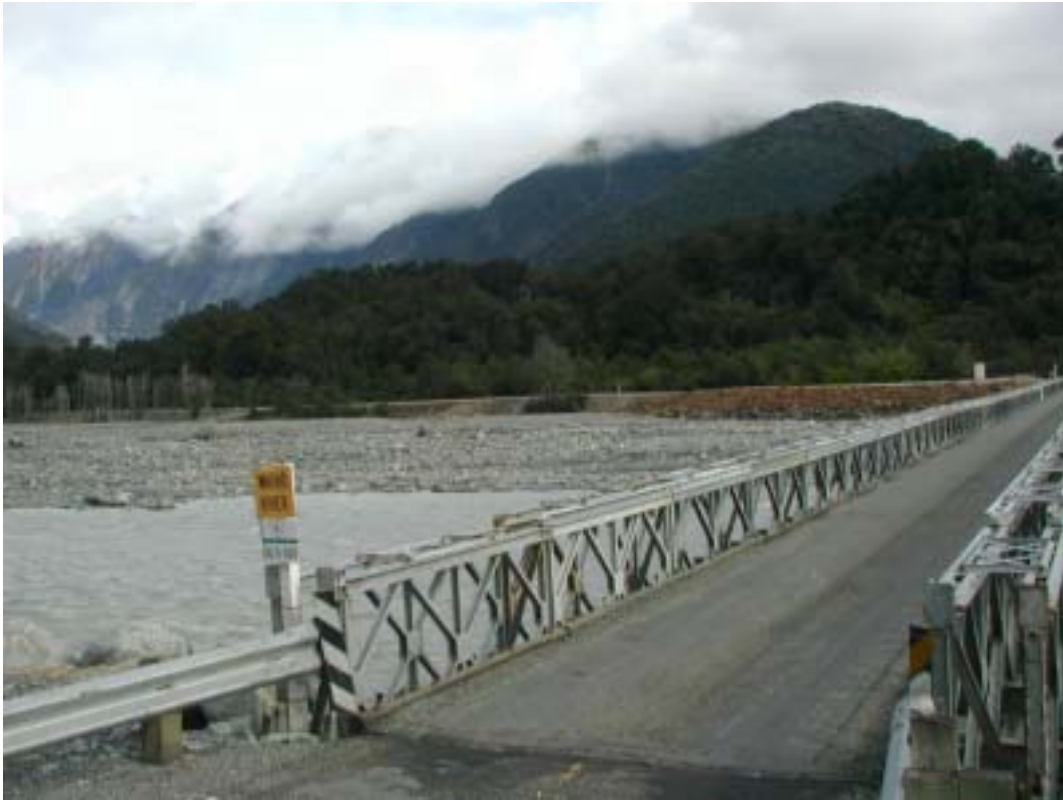
Figure 5.1: Glacier Access Road and SH6 bridge.
