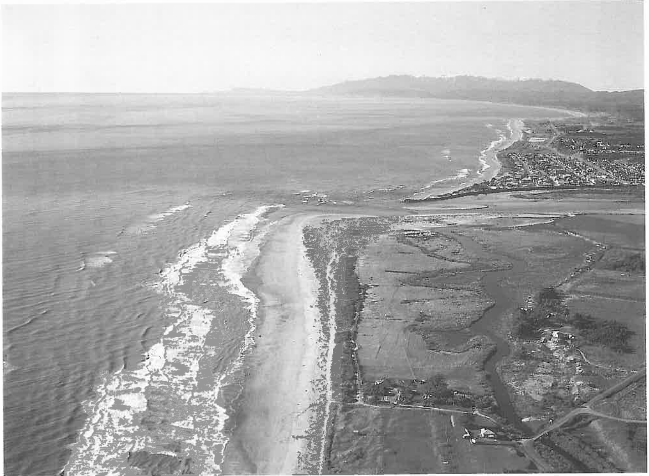
FIGURE 16: Photograph looking north towards Hokitika. Net (?) longshore drift direction is towards top of picture. Note the updrift-seaward-offset configuration of the Hokitika River mouth. Photo by J G Gibb, August 1984.
