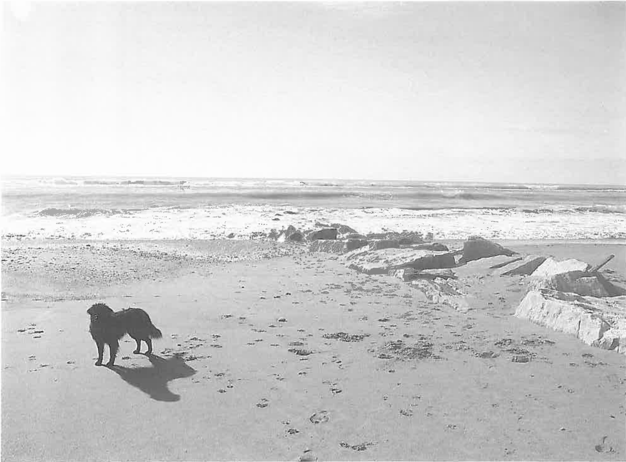
FIGURE 2: Photograph of rock groyne adjacent to Richards Drive. Sand has been trapped on the updrift (south) side to the left of the groyne raising beach levels and is bypassing northward through the structure. Photo by Paul McGahan, February 1987.
