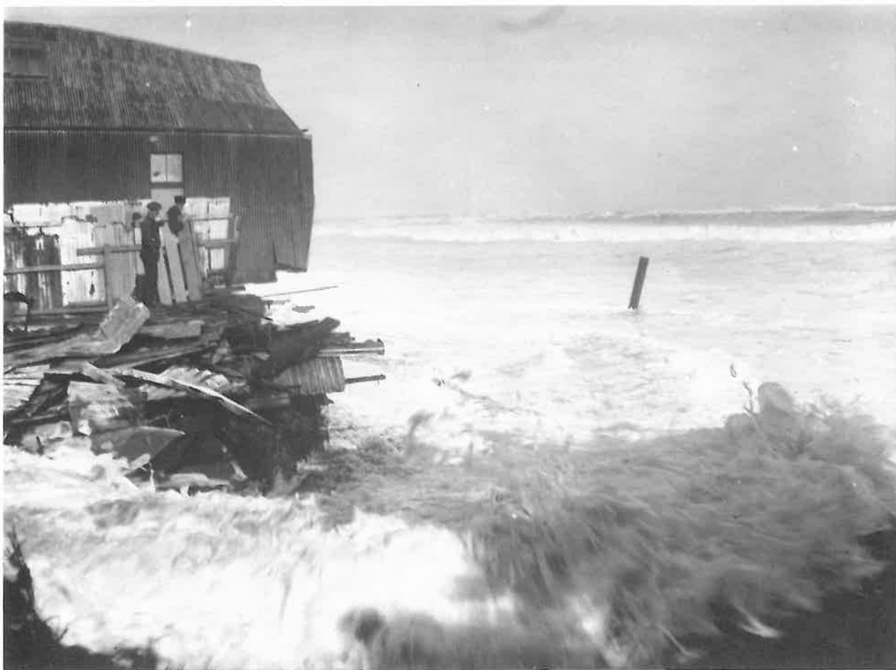
FIGURE 4: Photographs showing the impact of the 1913-1914 erosion phase on property and assets west of Revell Street near Weld Street. Despite such damage development has continued further seaward in the same area during periods of accretion. Top photo looking north; bottom photo looking south. Photos by Ben Thiern, April 1914, published by courtesy of the West Coast Historical Museum.
