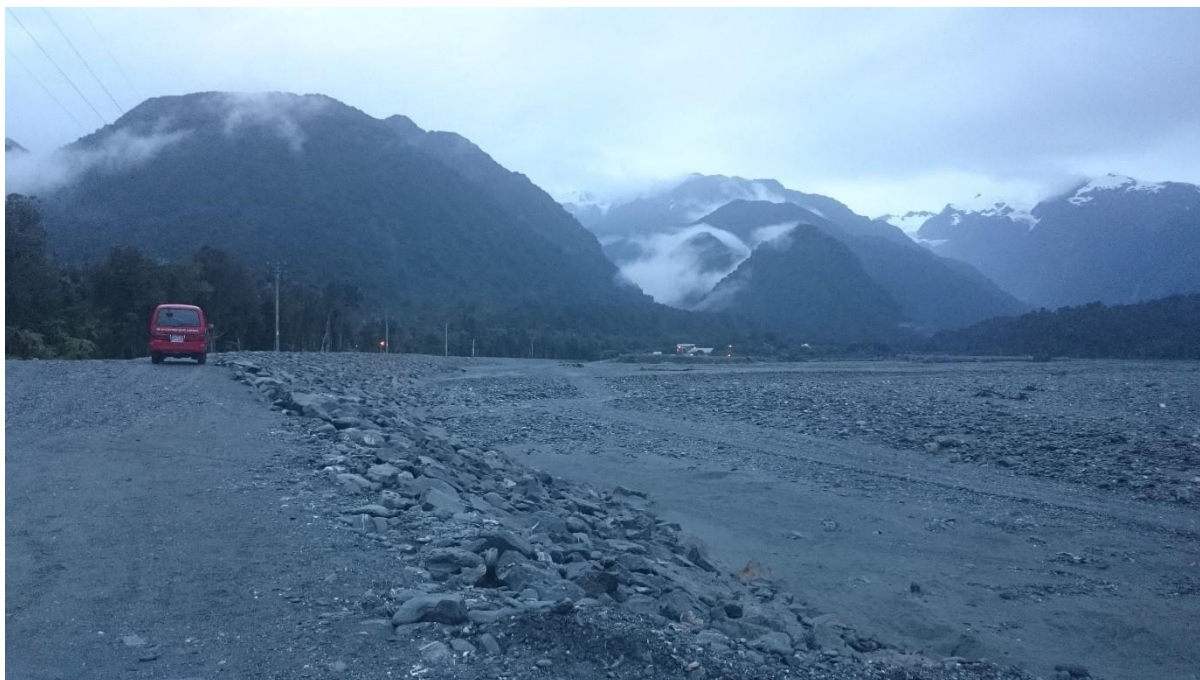
Figure 15-4: Power distribution network adjacent to the Waiho River
