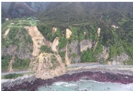
Figure 15-14: Landslides on to SH1 in the 14 November 2016 Kaikoura Earthquake
