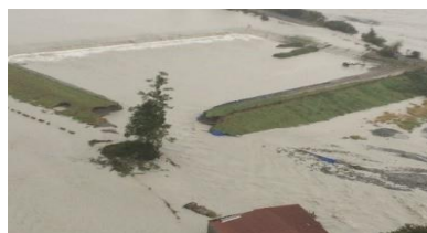
Figure 15-25: Flooding of the Waiho River in March 2016 impacting the wastewater treatment ponds (Opus, 2016)
