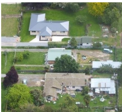
Figure 15-15: Shaking damage in Waiau in the 14 November 2016 Kaikoura Earthquake
