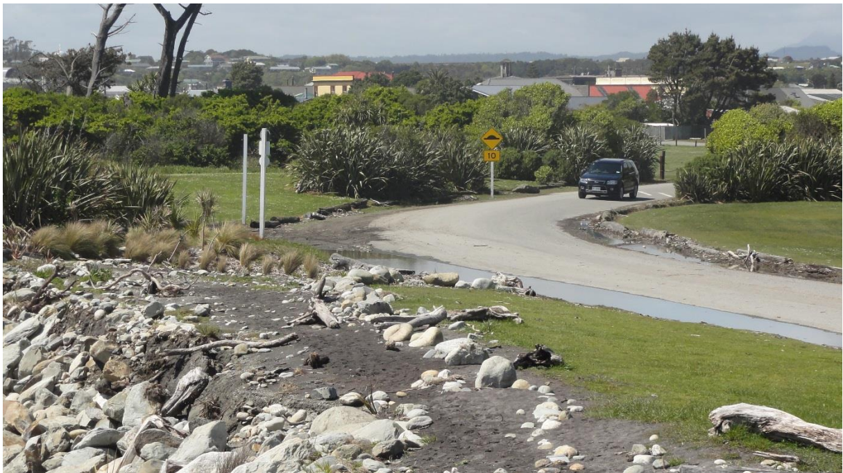
Figure 2-5: View east towards Sunset Point access road on 28 October 2015. Note driftwood litter and sand patches on grassy berm and beside road, placed by wave overwash.
