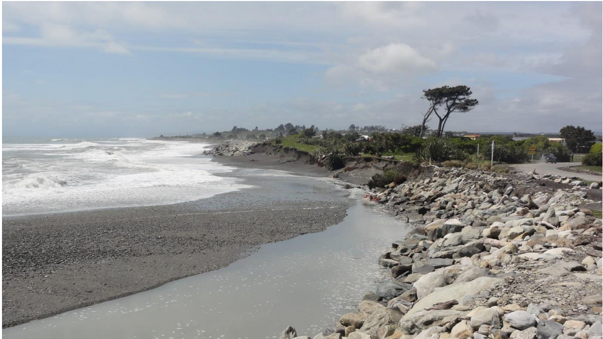
Figure 2-4: View north from “Tambo” at Sunset Point on 28 October 2015. Note terminus of foreshore-bar extending past Sunset Point, erosion in un-protected span of shore between rip-rap seawall segments, finer rock size and lower height of seawall adjacent to eroding section, and channel conveying swash to eroding section.
