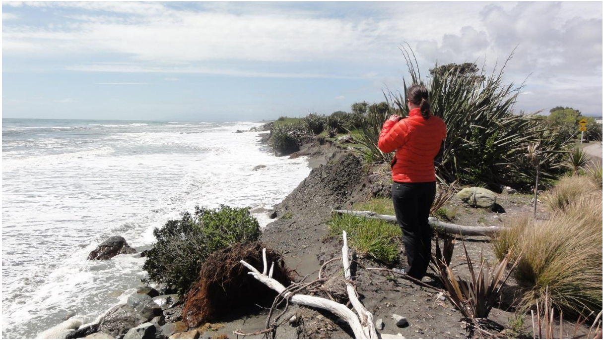
Figure 2-6: View north along eroding, unprotected span of foreshore between seawalls on 28 October 2015. Photo taken just north of “Tambo”.
