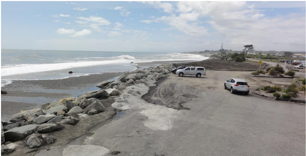
Figure 2-3: View north from Sunset Point lookout at Hokitika River mouth on 28 October 2015. Note beach/foreshore-bar in front of carpark and obliquely-breaking waves driving northward longshore transport.
