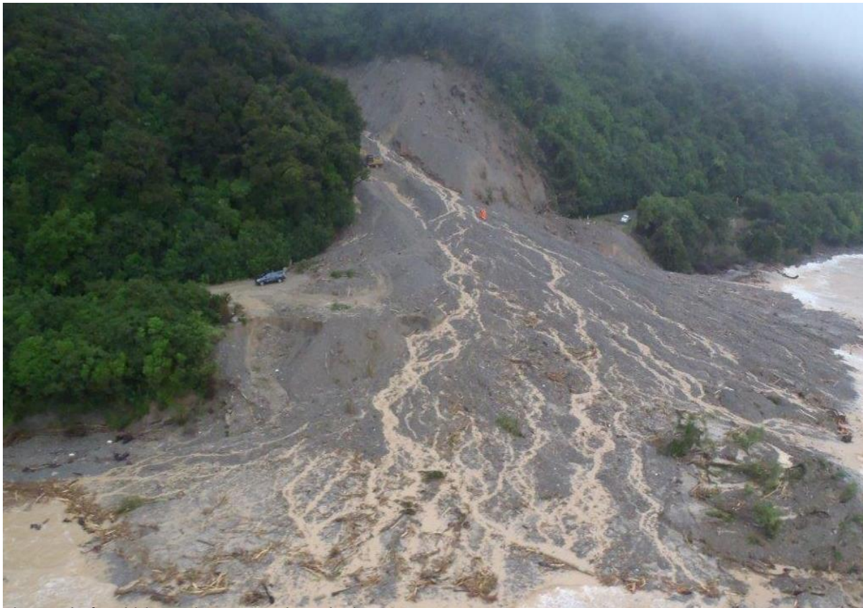
Photograph of Landslide at Jackson Bay, South Westland
