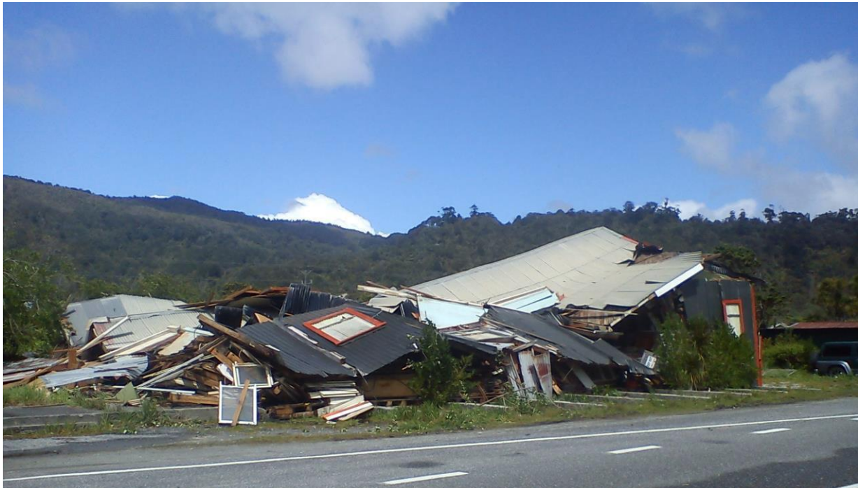
Photograph of damage caused by tornado Hector
